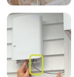
Do this again between the final connection point and the entry point to your home. In the event of rain or snow, this ensures water drips off the cable rather than into the unit or your home.
